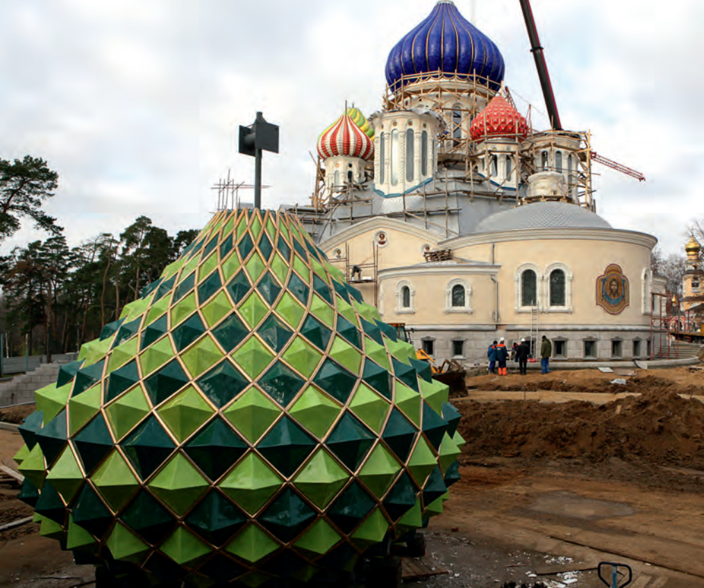
Installation of the ceramic cupolas of the Church of St. Igor of Chernigov (Novo-Peredelkino, Moscow), made at the Pallada workshop.
